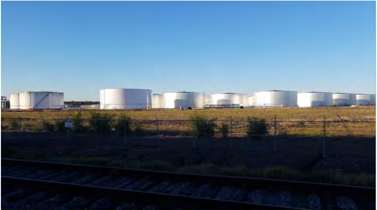
Photograph 7: WSLP-Maurepas Diversion, Pin Oak Oil Terminal tank farm, Garyville, LA, facing northwest.
