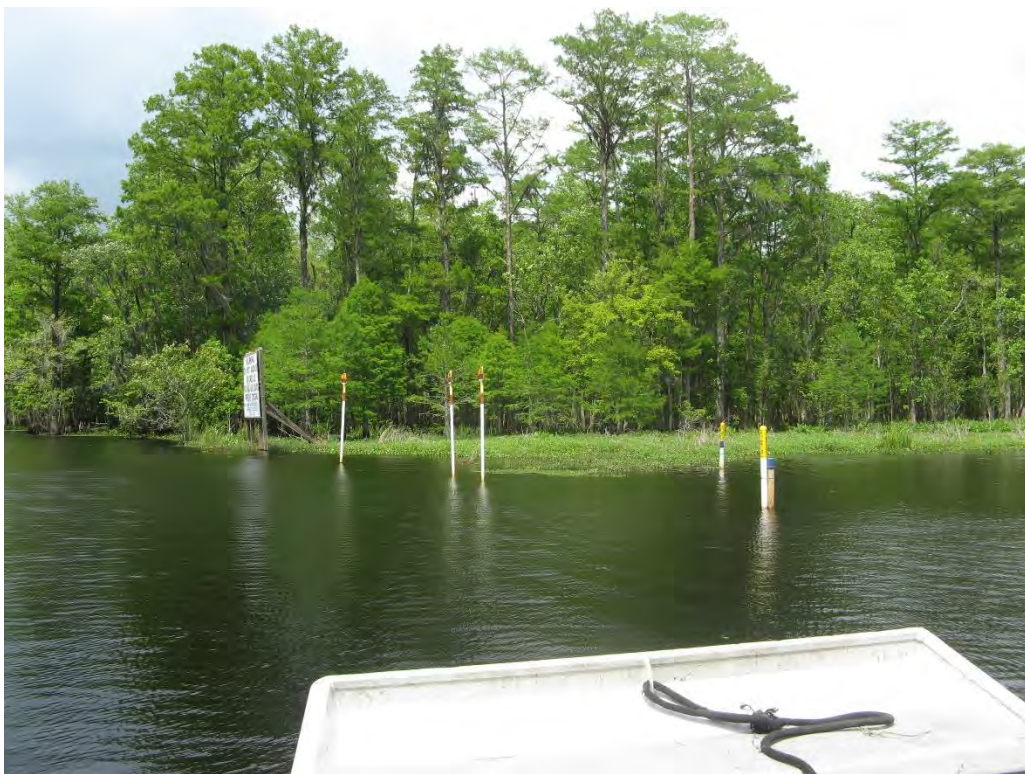
Photograph 4. Petroleum pipeline markers at intersection with Hope Canal in the Maurepas Swamp WMA, facing northeast.
